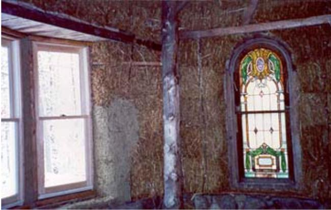
Inside view of straw bale studio showing straw bale construction and start of "cob" wall finish
